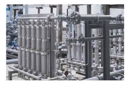
**Photo caption:** The picture shows membranes – a part of the helium purification facility in Mankota, Canada. (Source: The Linde Group).
