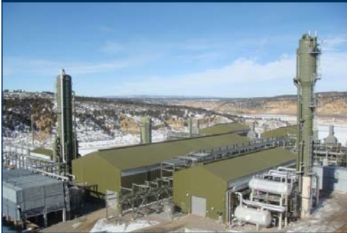
Natural gas processing plant
